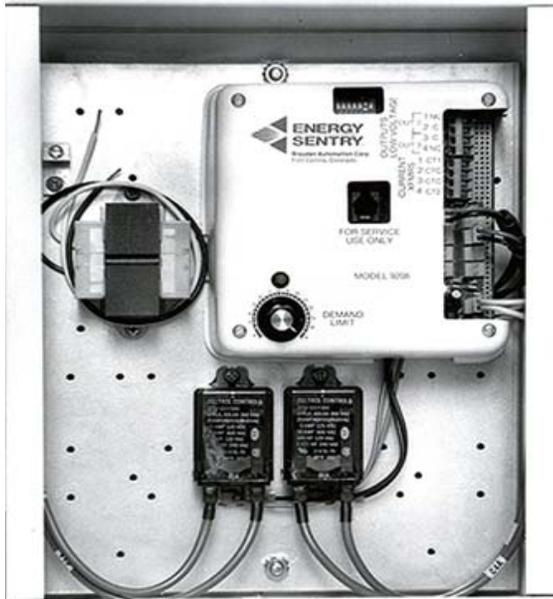
When this happens, the ENERGY SENTRY® system will give an audible warning (if the alarm is set to "on") that the limit is about to be exceeded. This means that you have a minute or two to turn off some of the uncontrolled loads to keep the meter from registering a higher KW than the control setting.
